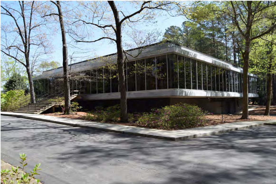
American Association of Textile Chemists and Colorists Headquarters Building (DH3963). View NW.
