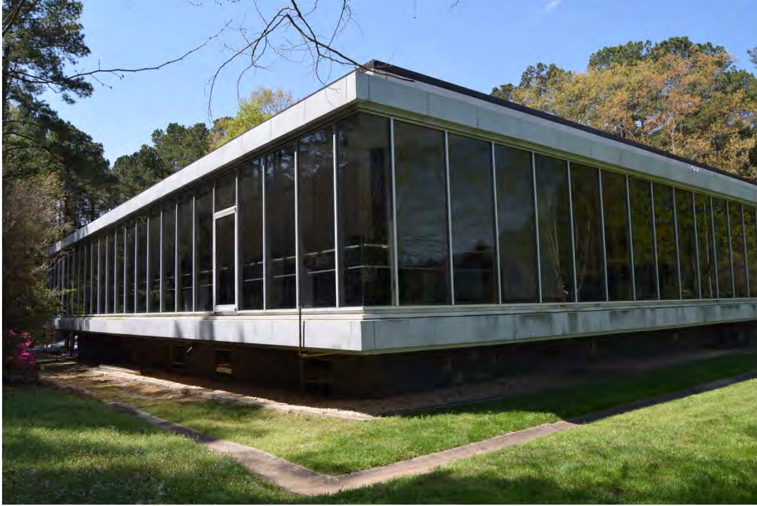
Rear and north elevations, American Association of Textile Chemist and Colorists Headquarters Building (DH3963). View SE.
