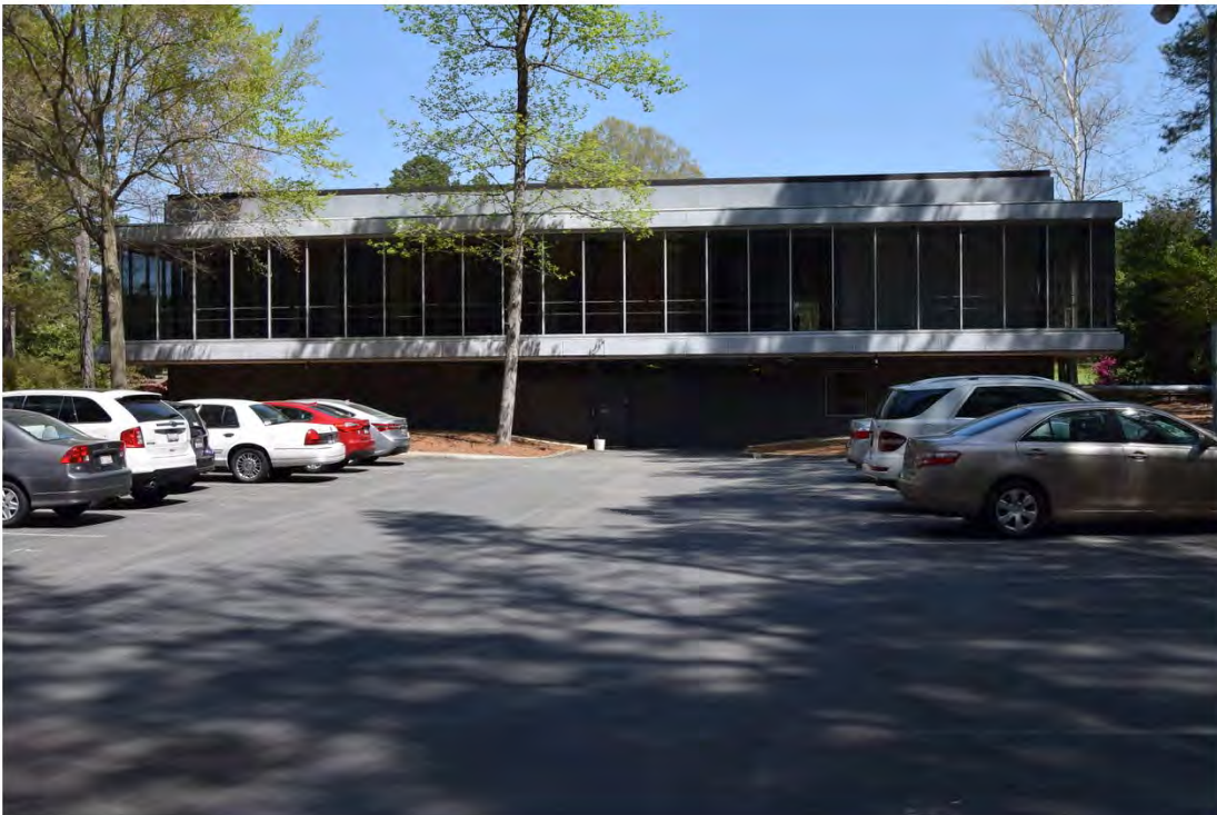
South elevation, American Association of Textile Chemist and Colorists Headquarters Building (DH3963). View N.
