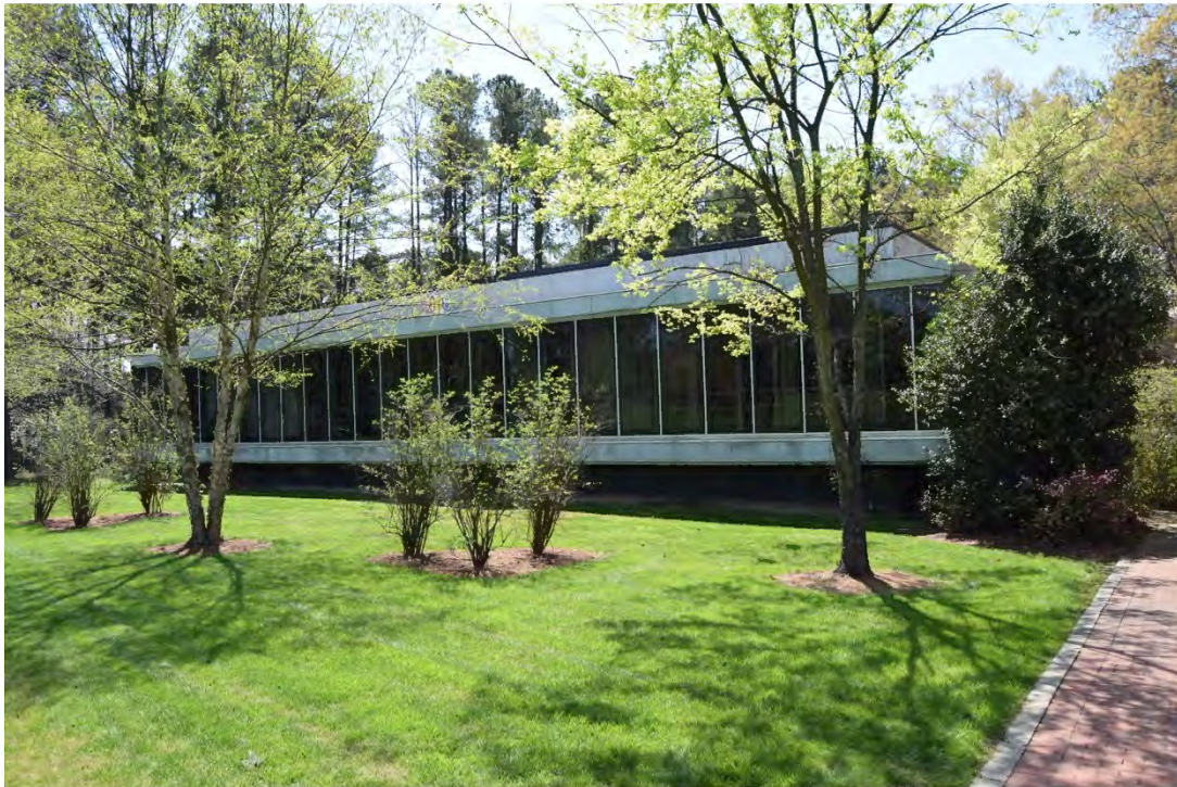
North elevation, American Association of Textile Chemist and Colorists Headquarters Building (DH3963).
